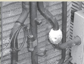
After one week CORROSION GRENADE has turned white due to galvanic corrosion. The corrosion attacked CORROSION GRENADE instead of expensive metal parts.
